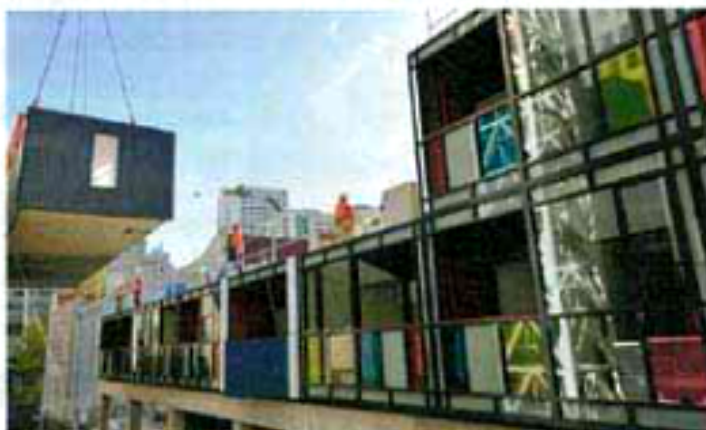
The United Building being put together in Albert Park, VIC
